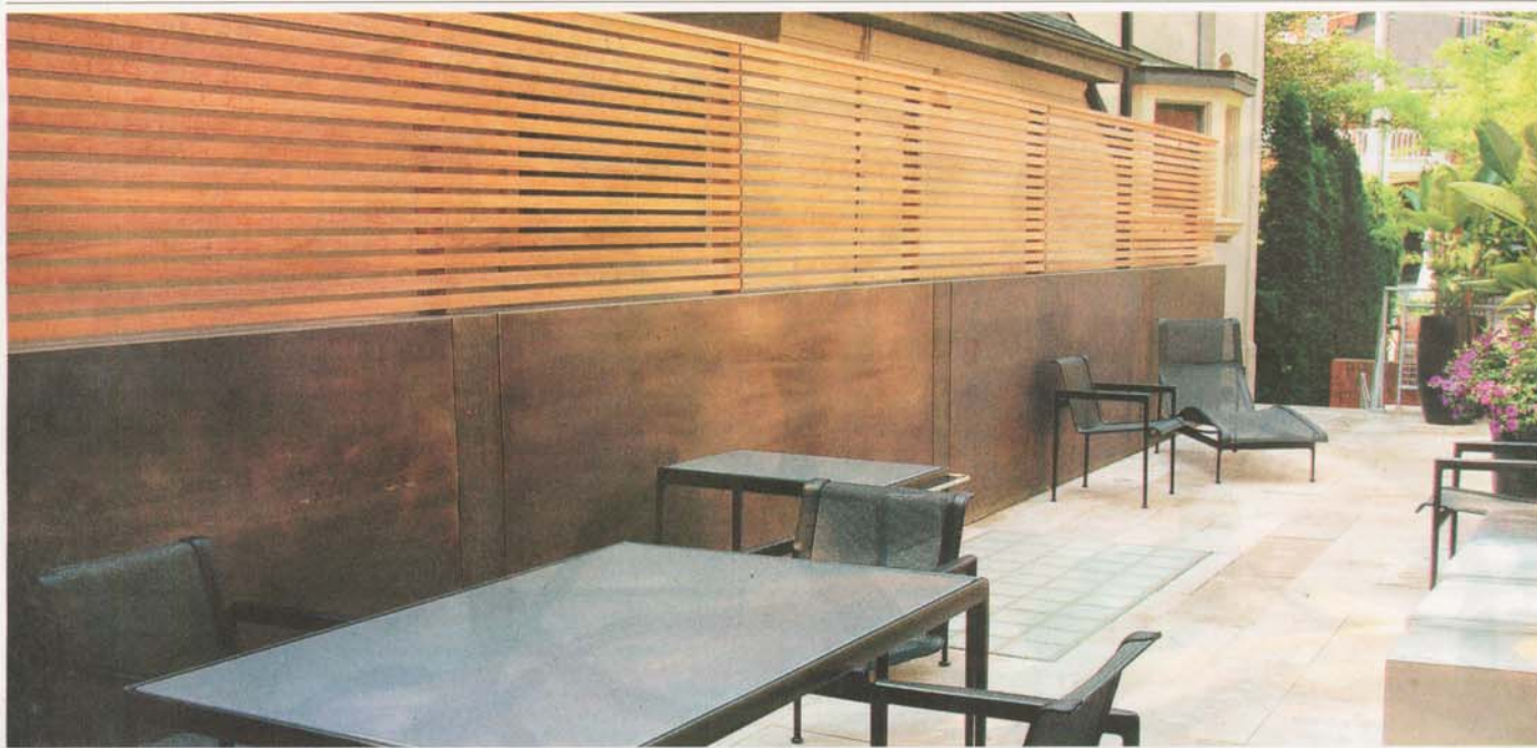
A wall of horizontal lpe wood slats lightens a base of Cor-ten steel in a garden by Janet Rosenberg and Associates. Both materials are extremely durable and will weather beautifully over time. JACKIE BEALE/JRA
