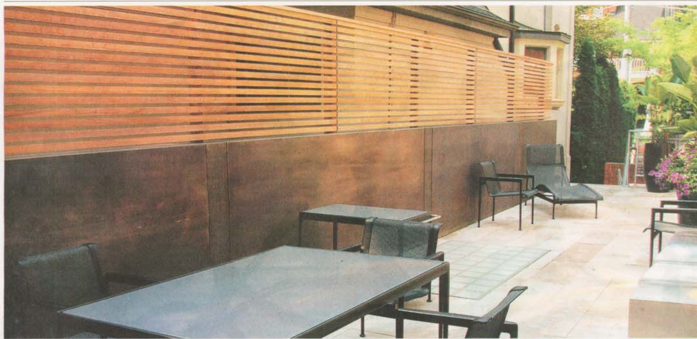
A wall of horizontal lpe wood slats lightens a base of Cor-ten steel in a garden by Janet Rosenberg and Associates. Both materials are extremely durable and will weather beautifully over time. JACKIE BEALE/JRA
